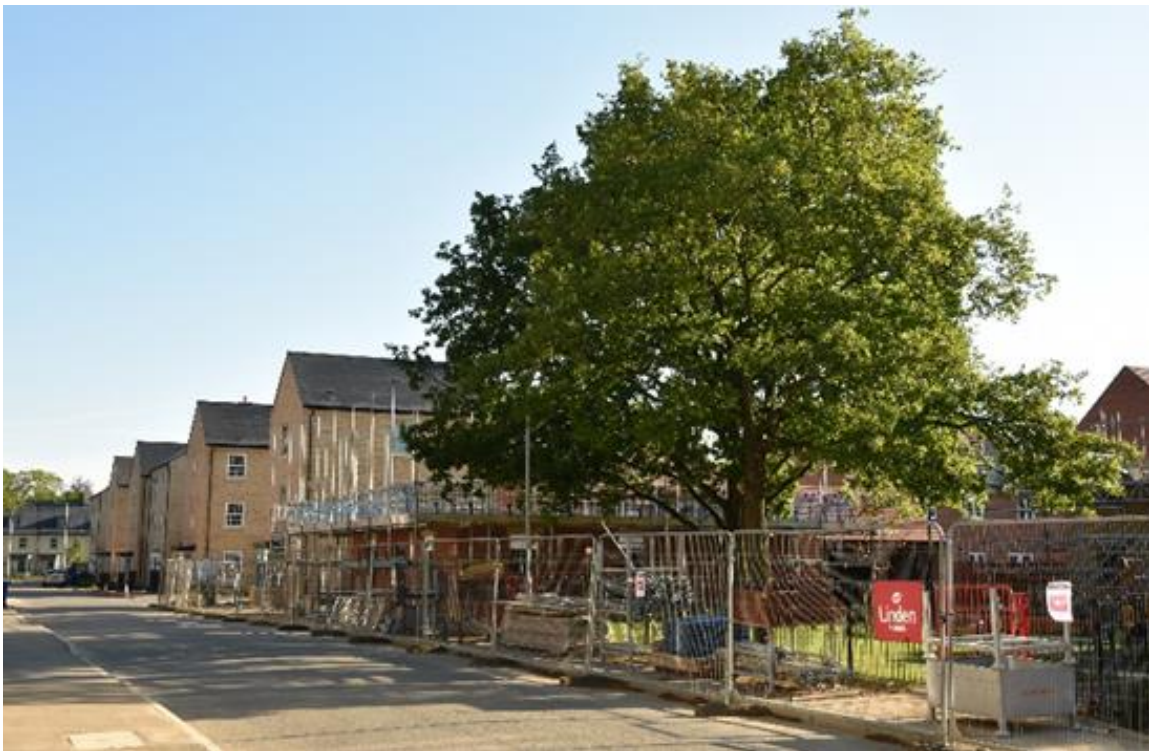
Forster Road, Brampton (HDC)
